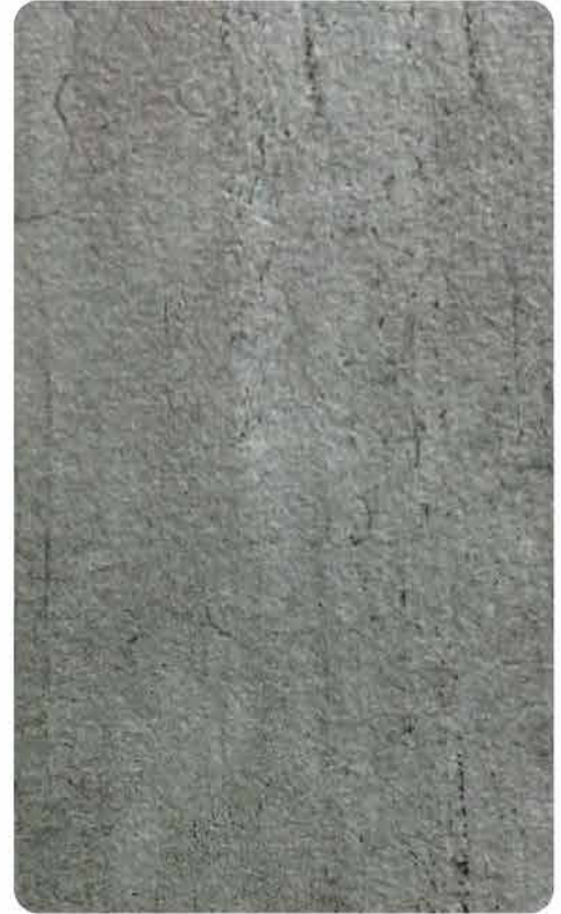
Concrete TH 1221 FC View
